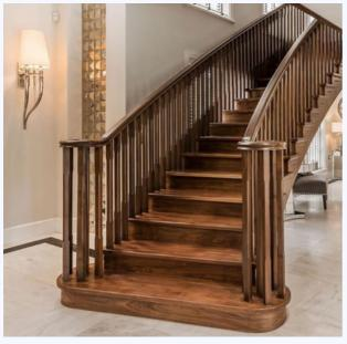
Here you will be able to see the profile of the steps climbing up the staircase, and as with the Closed String, this can be used in both traditional and contemporary projects for striking effect.
